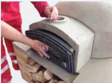
**7.** Push the door frame into the arch while the cement is still wet and drop the locking pin into position
