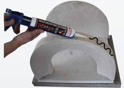
**3.** Place the front and run a bead of silicone over the top of the back and the front
