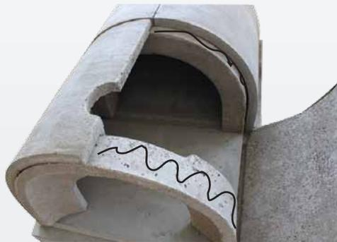
**5.** Run silicone on the top of the oven before placing the tops
