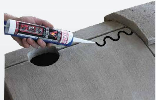
**6.** Finally seal underneath the chimney flange with silicone
