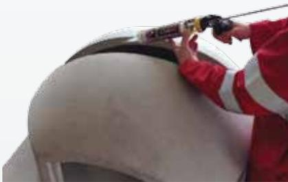
**4.** Place the front section and put heat resistant silicone on one of the faces to be joined
