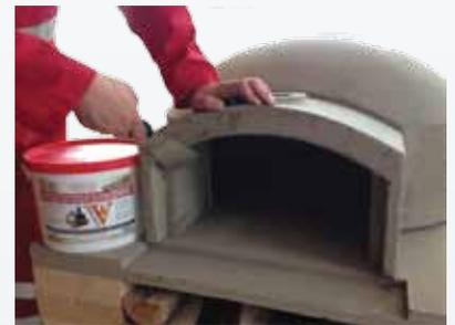
**6.** Trowel outdoor oven cement around the opening of the front arch
