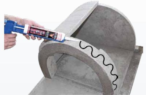
**3.** Place the front and back and run a bead of silicone over the top of the back and the front
