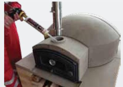
**9.** Put Heat Resistant Silicone around the top of the vent before dropping the flue into position
